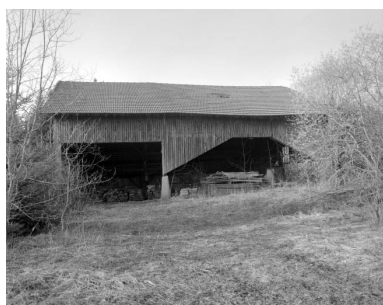
Magasin industriel. Phot. Yves Sancey IVR43_19983900032X
