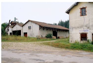
Atelier de fabrication. Phot. Yves Sancey IVR43_19973901472ZA
