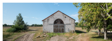
Vue de face. Phot. Pierre-Marie Barbe-Richaud IVR26_20195800606NUC4AQ
