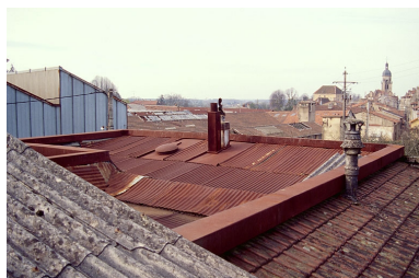
Toiture. Phot. Yves Sancey IVR43_19943900834ZA
