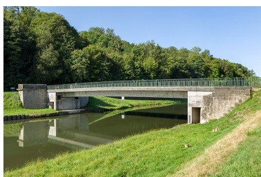
Pont de la D152 enjambant le canal. Phot. Sonia Dourlot IVR43_20157001557NUC2A
