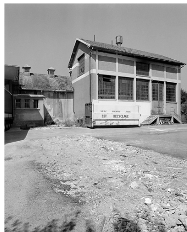
Chaufferie. Phot. Yves Sancey IVR43_20009000215X
