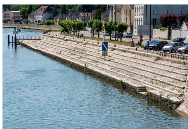
Les gradins. Phot. Jérôme Mongreville IVR43_20197000337NUC4A
