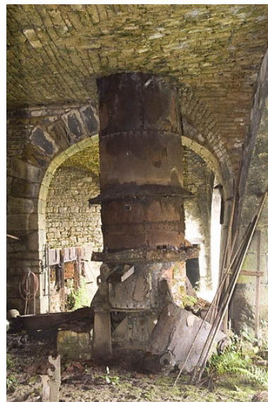
Cubilot ouest. Phot. Jérôme Mongreville IVR43_20087000961NUC2A
