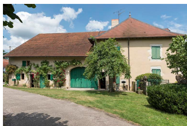
Façade principale Phot. Sonia Dourlot IVR43_20167001132NUC4A
