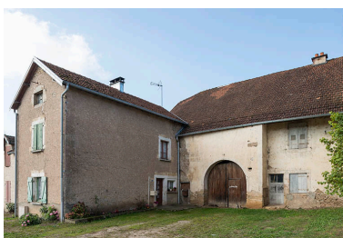
Ferme, Grande rue. Phot. Jérôme Mongreville IVR43_20167001611NUC4A
