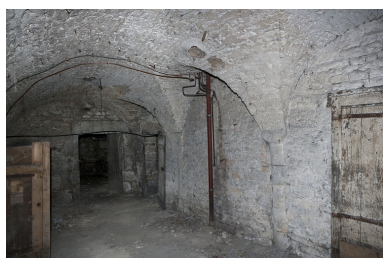
Logis principal, sous-sol : cave C. Phot. Yves Sancey IVR43_20112500715NUC2A
