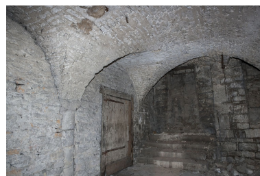
Logis principal, sous-sol : cave C. Phot. Yves Sancey IVR43_20112500714NUC2A
