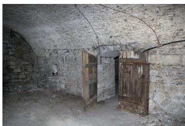
Logis principal, sous-sol : cave C. Phot. Yves Sancey IVR43_20112500713NUC2A
