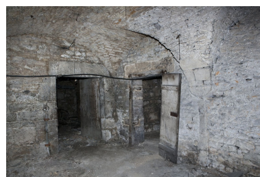
Logis principal, sous-sol : cave C. Phot. Yves Sancey IVR43_20112500717NUC2A
