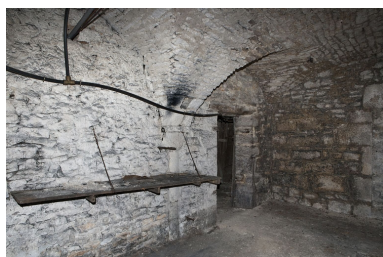
Logis principal, sous-sol : cave C. Phot. Yves Sancey IVR43_20112500712NUC2A
