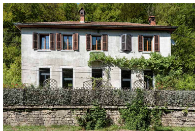
Façade antérieure. Phot. Sonia Dourlot IVR43_20192501465NUC4A
