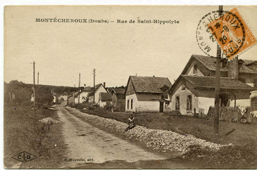
Montécheroux (Doubs) - Rue de Saint-Hippolyte, [1er quart 20e siècle]. IVR43_20192501146NUC4A
