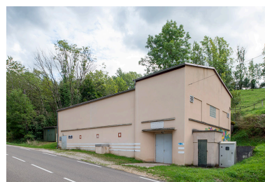
Station de stérilisation (1937), R.D. 472. Phot. Nicolas Waltefaugle IVR43_20253900255NUC4A
