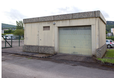
Garage. Phot. Sonia Dourlot IVR43_20142501056NUC2A
