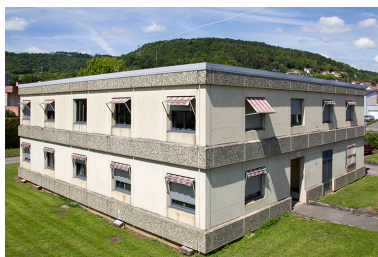
Angle sud des logements. Phot. Sonia Dourlot IVR43_20142501059NUC2A
