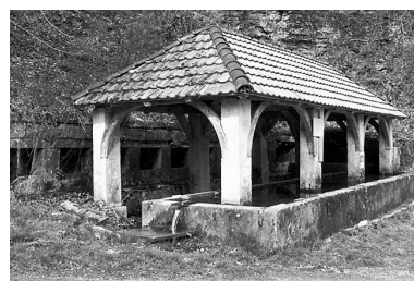
Fontaine-lavoir Phot. Bernard Lardière IVR43_19829000314Z
