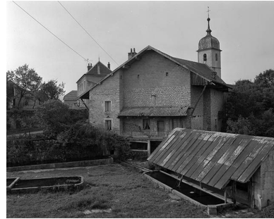
Elévation du logis. Phot. Yves Sancey IVR43_19802500881X
