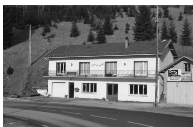
Logement patronal. Phot. Laurent Poupard IVR43_19913901612Z
