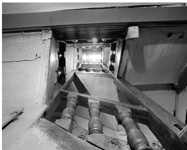
Escalier. Phot. Jérôme Mongreville IVR43_19872500500X
