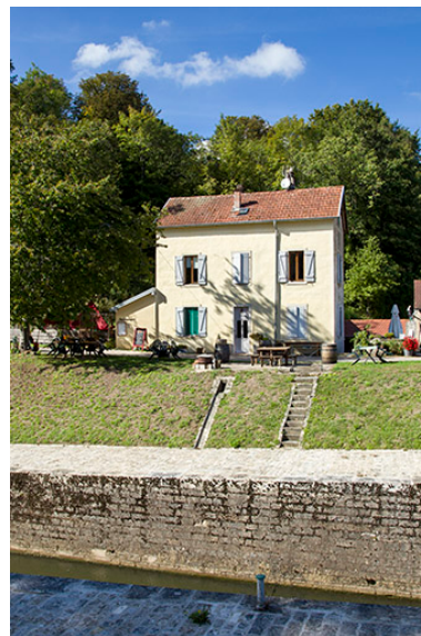
La façade antérieure. Phot. Sonia Dourlot IVR43_20157001002NUC2A
