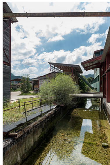
Scierie Boillot : le canal. Phot. Sonia Dourlot IVR43_20172501067NUC4A
