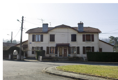
Façade antérieure. Phot. Marc Loukachine IVR43_20122500263NUC2A
