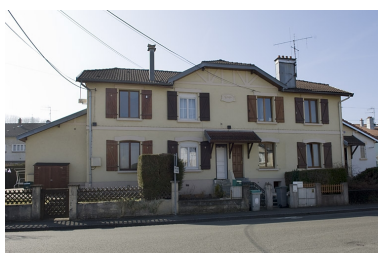
Façade antérieure. Phot. Marc Loukachine IVR43_20122500264NUC2A
