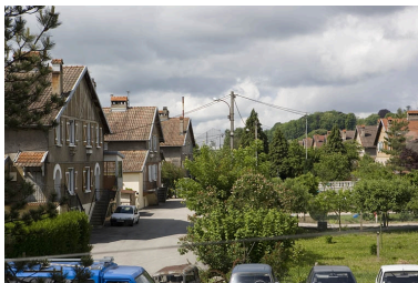
Cité Lehmann. Place de Chemontey.
