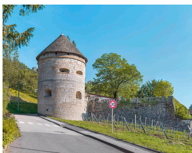
Elévation nord. Phot. Thierry Kuntz IVR43_20223900614NUC4A
