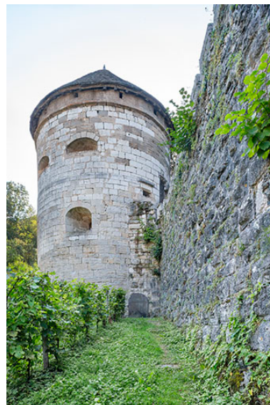
Elévation ouest. Phot. Jérôme Mongreville IVR43_20243900861NUC4A
