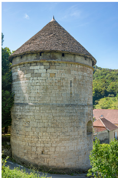
Elévation nord. Phot. Jérôme Mongreville IVR43_20243900849NUC4A
