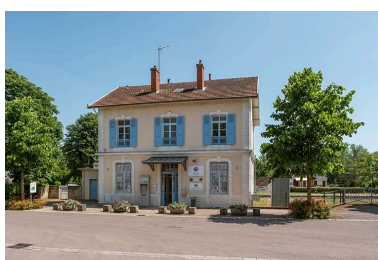
Façade nord. Phot. Pierre-Marie Barbe-Richaud IVR26_20212100001NUC4A
