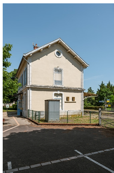
Façade ouest. Phot. Pierre-Marie Barbe-Richaud IVR26_20212100002NUC4A
