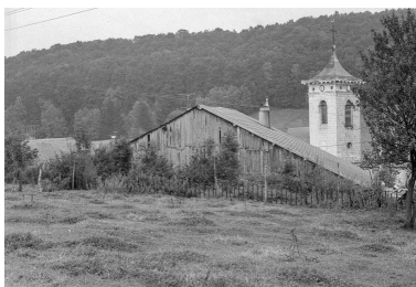
Façade postérieure. Phot. Gilbert Poinot IVR43_19752501366Z
