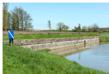
Digue ferroviaire. Phot. Sonia Dourlot IVR43_20167000313NUC4A
