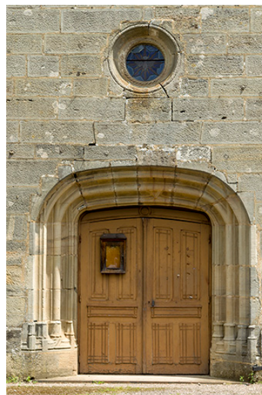
Portail Phot. Sonia Dourlot IVR43_20157001350NUC2A
