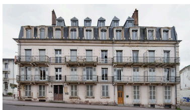
Façade nord. Phot. Jérôme Mongreille IVR43_20207000619NUC4A
