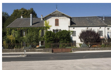
Logement patronal. Phot. Jérôme Mongreville IVR43_20067000862NUCA
