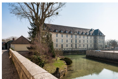
Dole, lycée Charles Nodier : internat. Phot. Jérôme Mongreville IVR43_20143900249NUC4A
