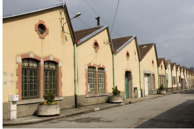
Pignons de sheds. Phot. Jérôme Mongreville IVR43_20067000146NUCA
