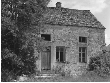
Façade principale. Phot. Jean-Luc Duthu IVR26_19748901128V
