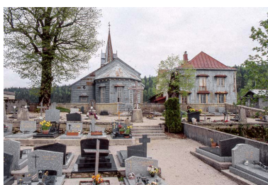
Chevet. Phot. Yves Sancey IVR43_19993900233ZA
