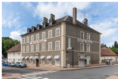
Façade sud et façade est. Phot. Pierre-Marie Barbe-Richaud IVR26_20217100241NUC4A
