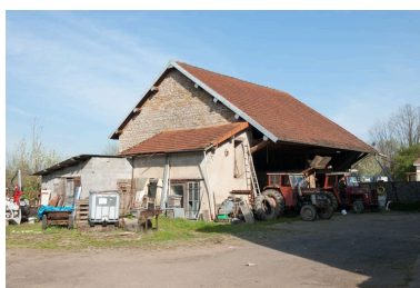
Hangar agricole. Phot. Jérôme Mongreville IVR43_20102500631NUC4A
