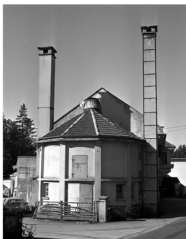
Chaufferie. Phot. Yves Sancey IVR43_19973901383X
