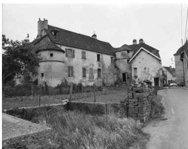
Façade ouest. Phot. Yves Sancey IVR43_19813900177X
