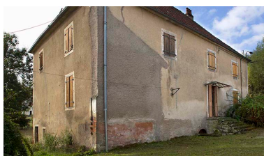
Façade postérieure. Phot. Sonia Dourlot IVR43_20157000601NUC2A
