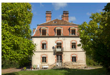
Façade sud. Phot. Sonia Dourlot IVR43_20157000679NUC2A
