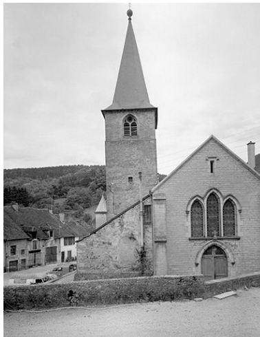
Façade antérieure. Phot. Yves Sancey IVR43_19853900230V
