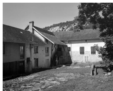
Logements. Phot. Yves Sancey IVR43_19973901407X
