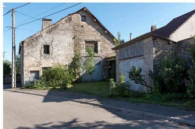
Façade antérieure. Phot. Sonia Dourlot IVR43_20177000973NUC4A
