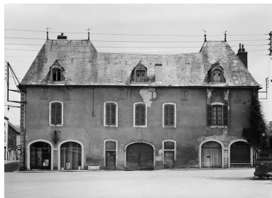
Façade principale. Phot. Jean-Luc Duthu IVR26_19802100161V
