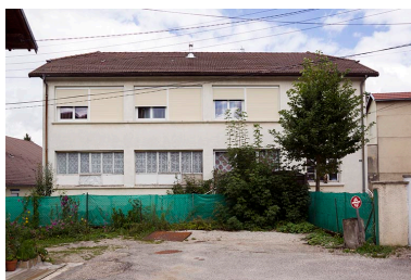
Façade antérieure. Phot. Yves Sancey IVR43_20132501788NUC2A
