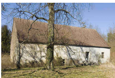
Logement patronal. Phot. Jérôme Mongreville IVR43_20097000173NUC2A
