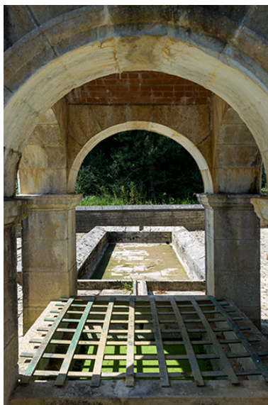
Puits. Phot. Sonia Dourlot IVR43_20167001853NUC2A
