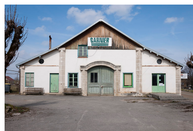
Mur-pignon est. Phot. Jérôme Mongreville IVR43_20162500220NUC4A
