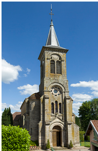
Façade principale. Phot. Sonia Dourlot IVR43_20157001030NUC2A
