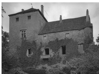
Façade postérieure. Phot. Michel Rosso IVR26_19802100598V
