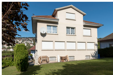
Façade postérieure. Phot. Sonia Dourlot IVR43_20162501282NUC4A
